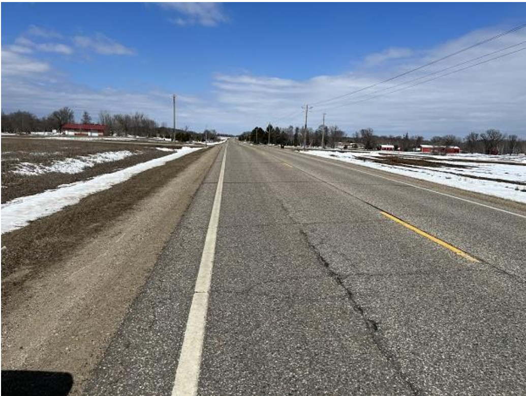
Looking north down County 11
